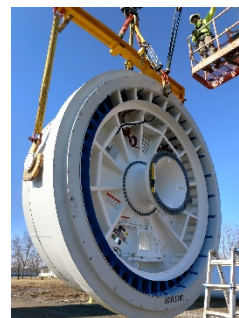
Turbine Generator being lifted using two vertical slings.
