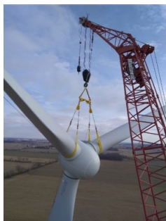
Rotor assembly being lifted using a double-basket configuration.
