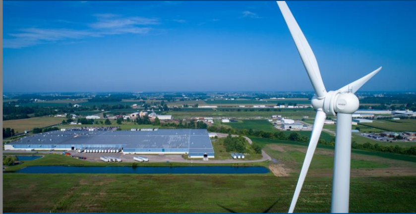
One Power Wind for Industry project - Ottawa, OH
