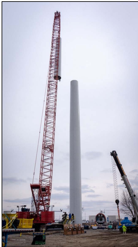
Figure 1: Construction of turbine tower
