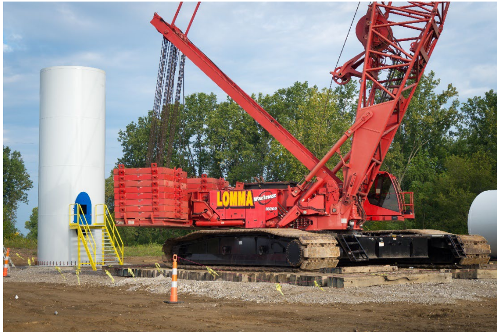
A crane mat in use
