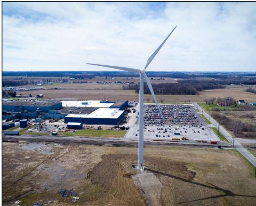
An operating Wind for Industry® turbine.
