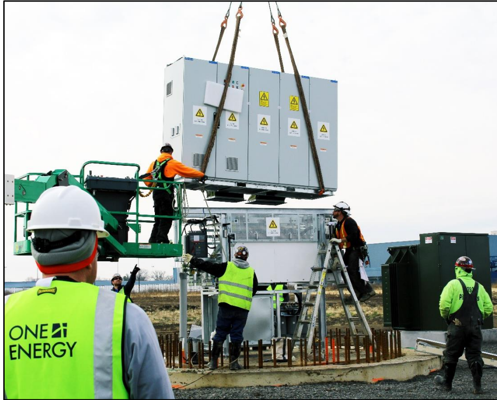
The interior electrical cabinets of the turbine are installed.
