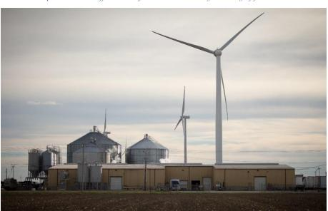
Here, you can see that the turbine in the foreground is yawed to face away from the camera; the turbine in the background is yawed to face the left of the picture. This difference in yaw can be caused by a variety of factors.
