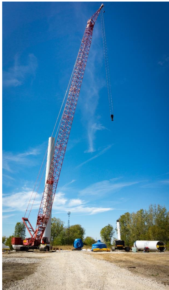
A crane mat in use
