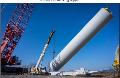
A tower section being tripped.
